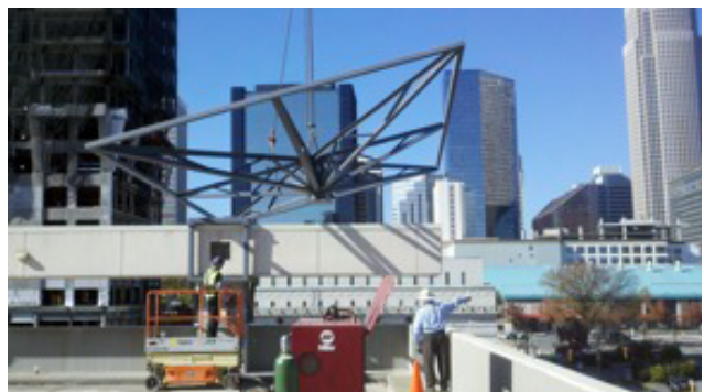
A crane lifts the structure that will support the solar panels into place.
