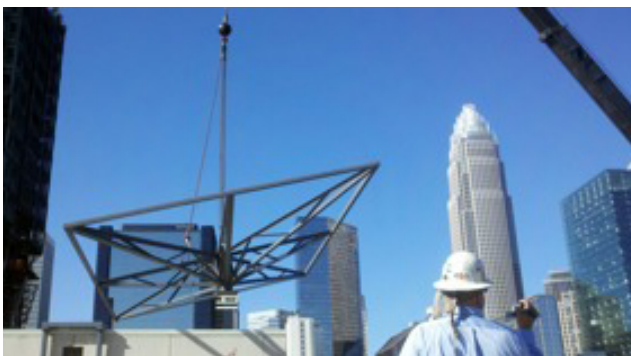
A crane lifts the structure that will support the solar panels into place.
